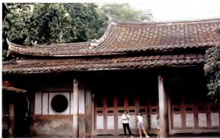
Fig. 8 Sanqing Dian (Hall of the Three Purities), the main hall at the Northern Song dynasty Xuanmiao Guan, constructed in 1016, in Putian, Fujian province.
